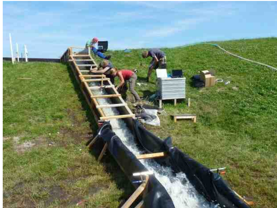
DredgDikes project, Rostock (Germany)
